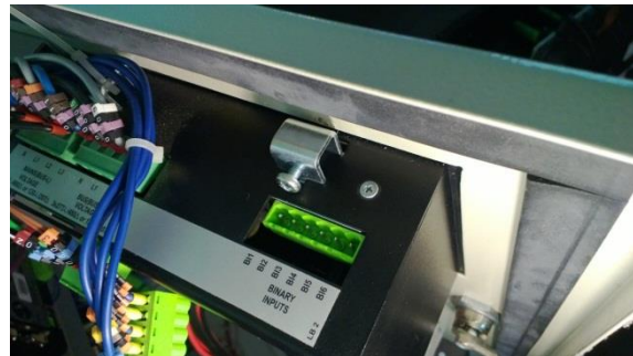
Tighten as required to fix the controller in the position
